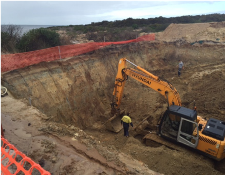
*Pump Station construction commenced in March 2016
