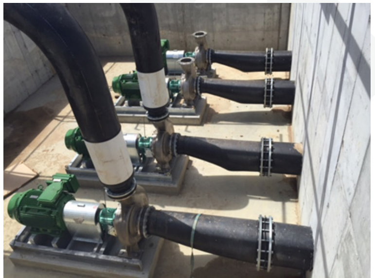
*Pump Station completed and first two pumps up and running December 2016
