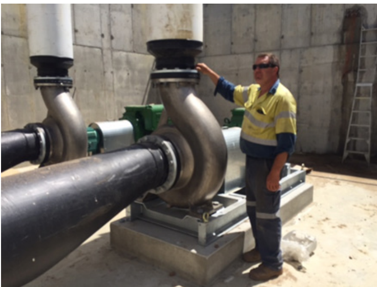
*Andrew Christian of Kasandi inspecting the pumps prior to first start up
